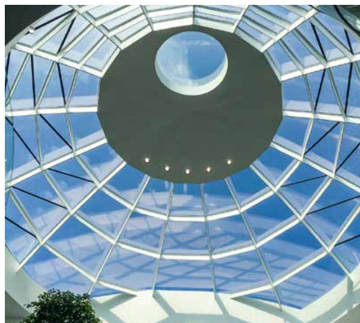
Office building - Bad Sankt Leonhard, AT
